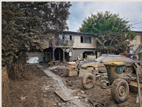
Thousands of homes in north NSW were damaged by the floods
