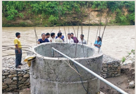
Connecting the solar powered irrigation pump to the water source
