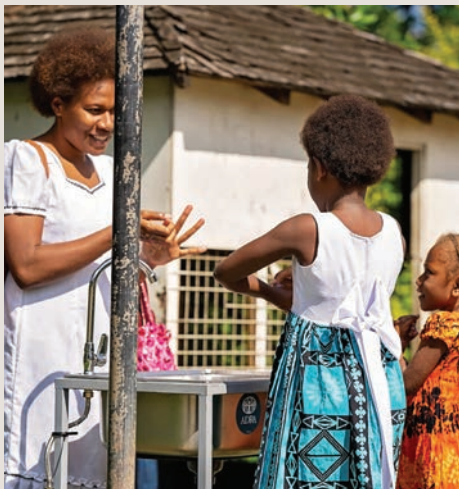
Sinks installed in churches in Vanuatu
